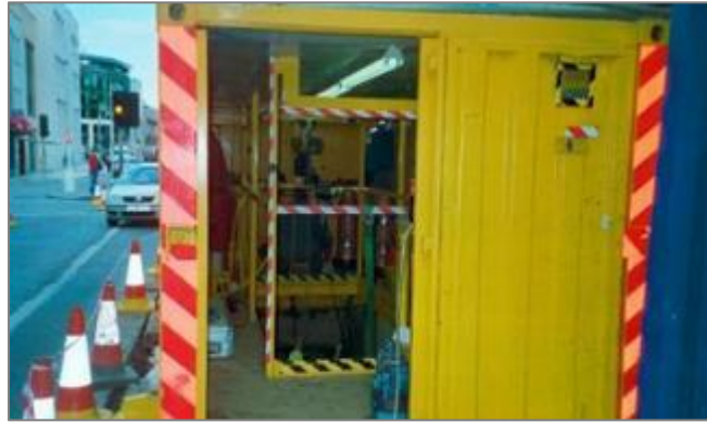
Figure 11 - HV cable jointing container
