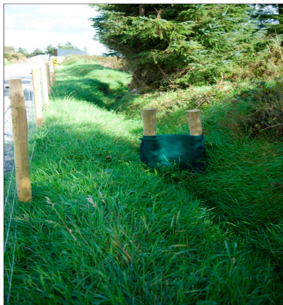
Image 4-1: Silt trap across grassed swale
