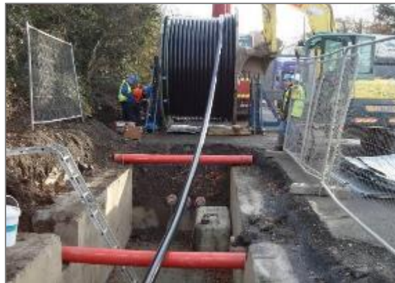
Figure 10 - HV cable pulling procedure (Drum set-up example)
