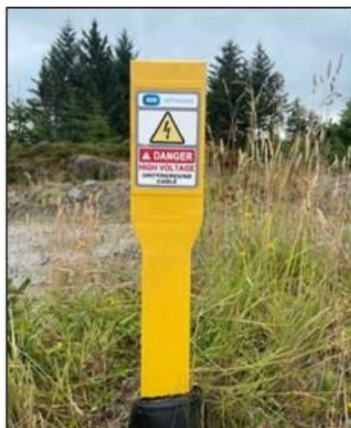
Figure 6 - EirGrid Marker Post
