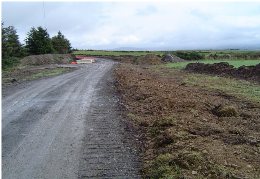
Image 4-3: Backfill over cable trench
