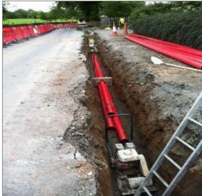
Figure 2 – Example of 110kV Underground Duct Installation
