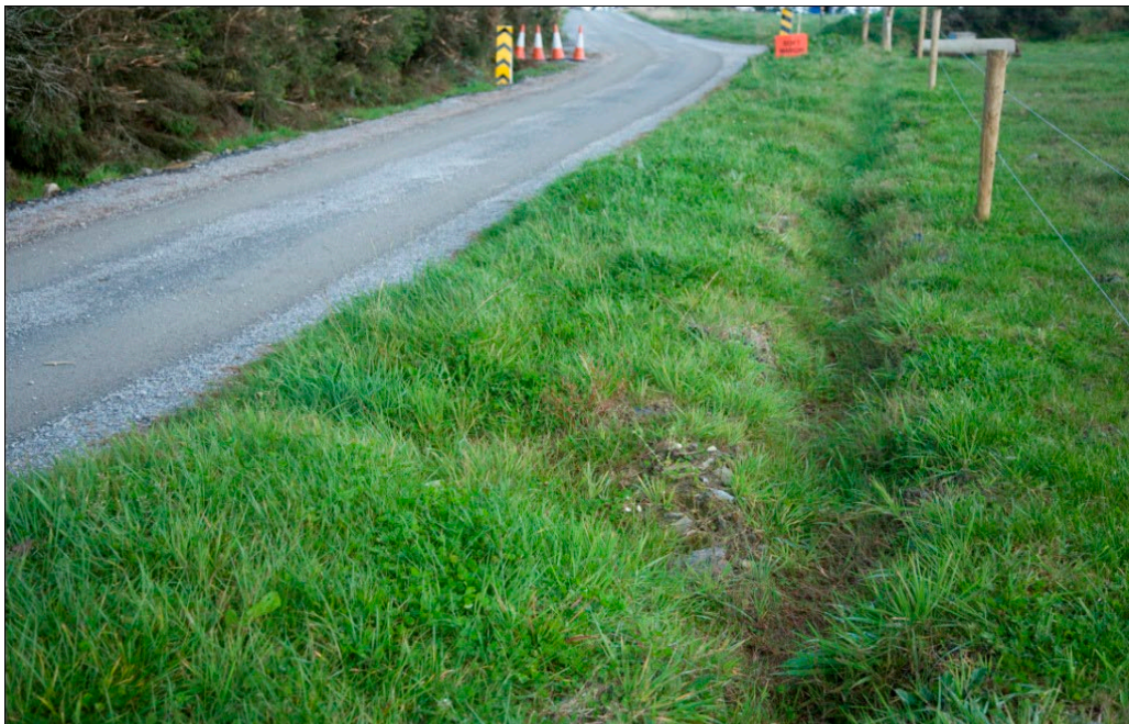
Image 2-2: Grassed swale along access track
