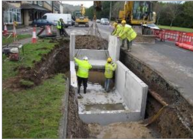
Figure 9 – Example of Joint Bay under construction (pre-cast)
